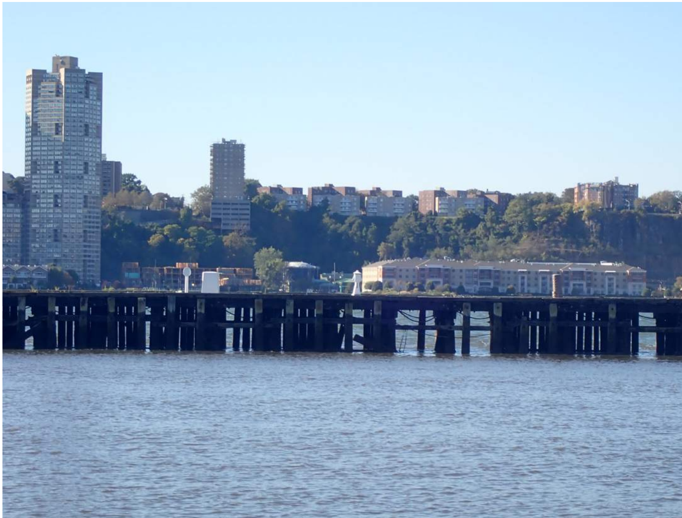
1 - View Looking West at Wave Screen
