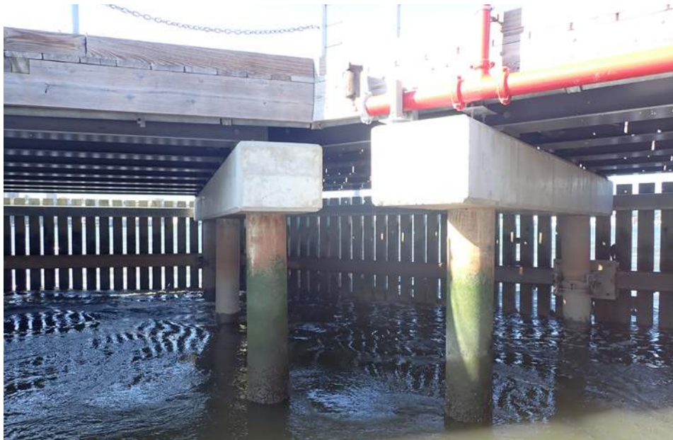
Steel Piles & Concrete Pile Caps
